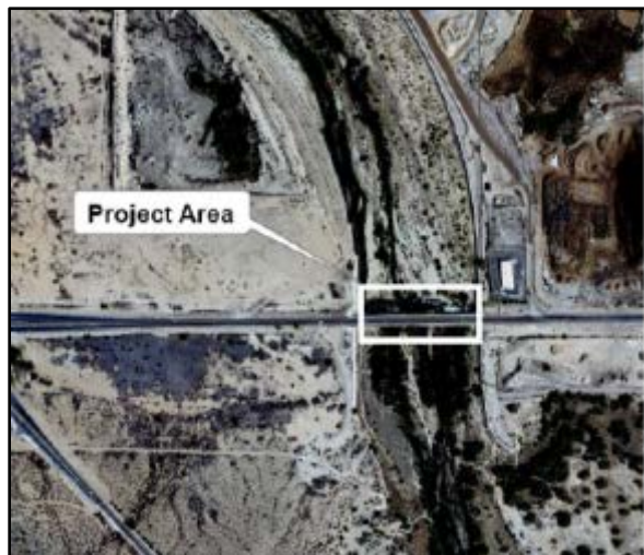
Figure 1. Ina Road Bridge over the Santa Cruz River, Marana AZ
