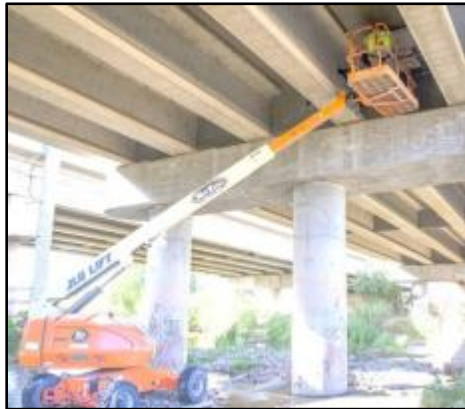
Figure 3. Installation of MODERNBAT © box under Cortaro Rd. Bridge
