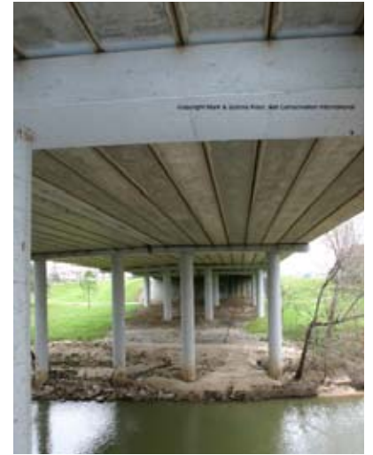
Waugh Street Bridge.
