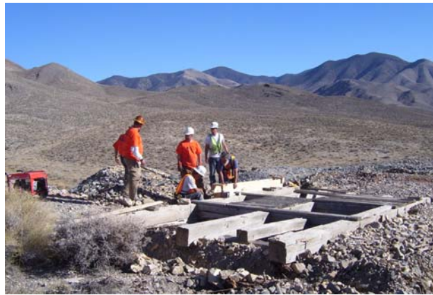
Figure 3. Construction of a bat gate near Gabbs, Nevada
